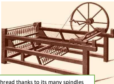
...y (1764) provided more thread thanks to its many spindles
